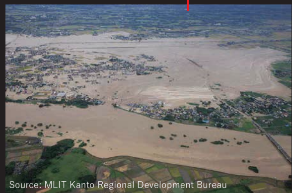
Photo 4: Point of embankment destruction (10 Sep 2015 around 15:00)
