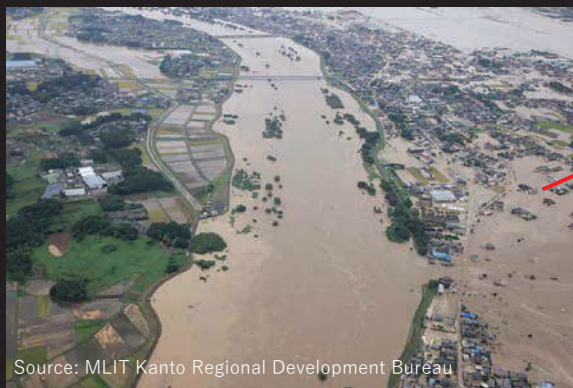
Photo 3: Point of embankment destruction (10 Sep 2015 around 15:00)
