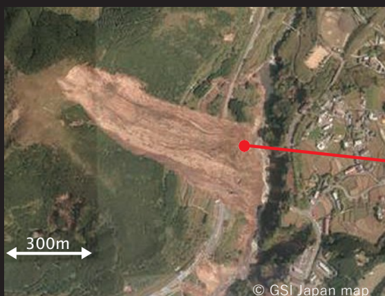
Photo 1: Vicinity of the Great Aso bridge after disaster (aerial photo) (16 Apr 2016)
